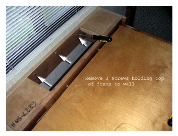
6. Remove the three screws holding bottom of cabinet frame to the wall.
